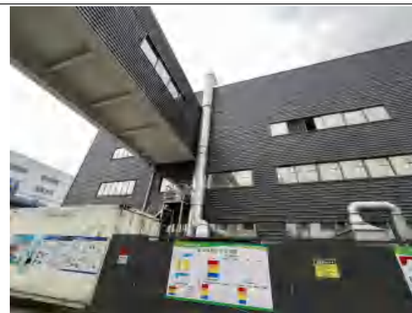
废气排放口 2DA001
